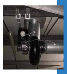
ATEX Polypropylene Fans Specifications Zone 2, EEX-d motor Category 3 gas explosion group IIB & IIA Temperature Class T4 - 135°C maximum surface temp of the motor, 40° ambient air temperature. Learn more ATEX Concepts here.
